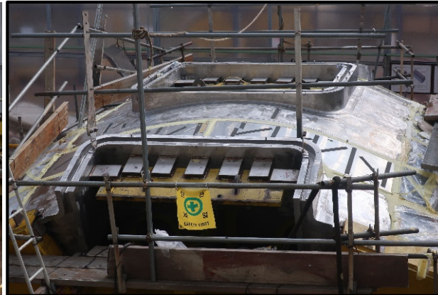
Poloidal Segment #3 (PS3): Outer Shell Welding Assembly
