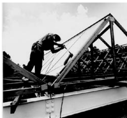
Dedication of the nation's largest solar heating and cooling system, currently in operation, took place November 26, 1975, at the George A. Towns Elementary School in Atlanta, Georgia. Solar collector panels mounted on the roof are pictured during construction.
