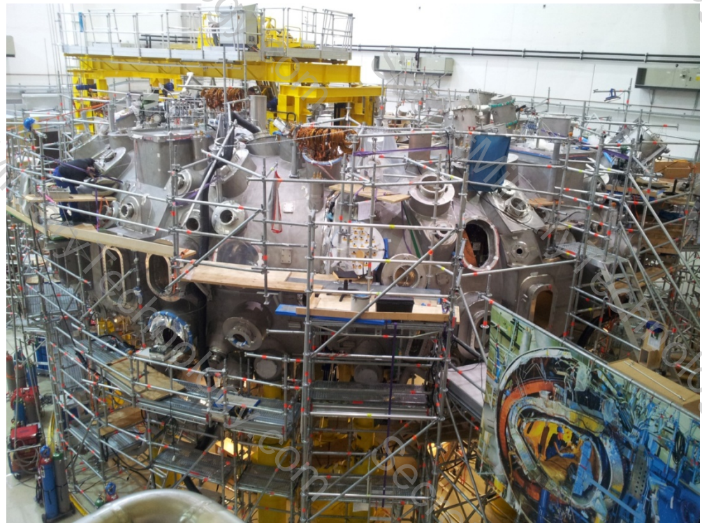
W7-X stellarator construction is proceeding. Completion in late 2014
