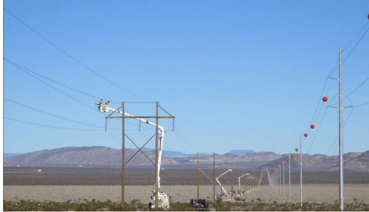
Crews working on the 138 kV Power Transmission System Replacement Project at NNSS
