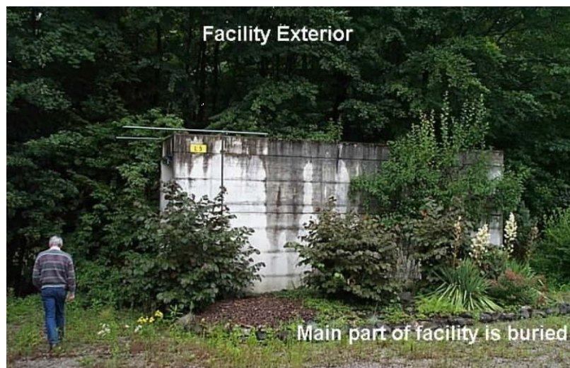
Figure 1. The exterior view of the underground Spiez test-bed facility.
