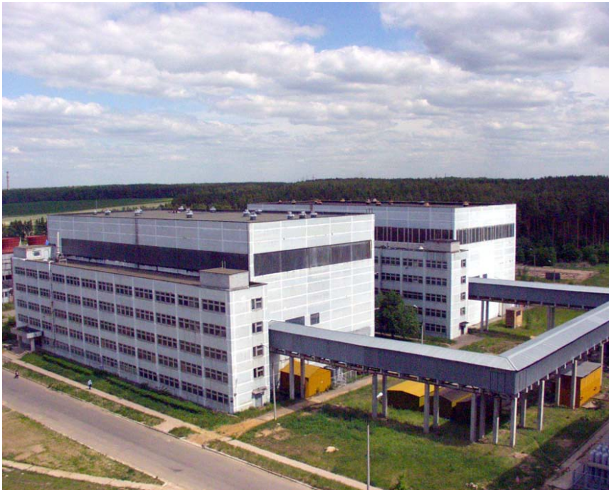
Buildings with 4 generators
