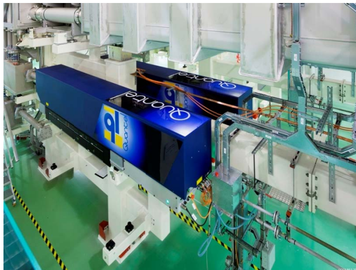
Figure V.2: PreAmplifier Module in the North-East Laser Bay
