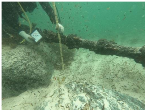
Nearshore split pipe cable protection inspection
