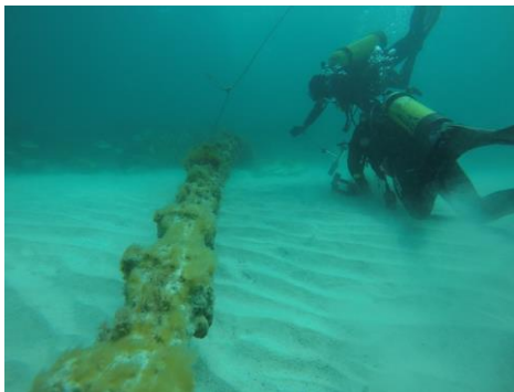
Nearshore split pipe cable protection inspection
