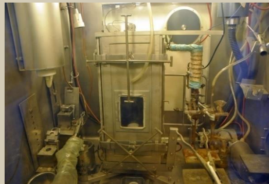
Hot Cell-1 Heating and Evaporation of I-131
