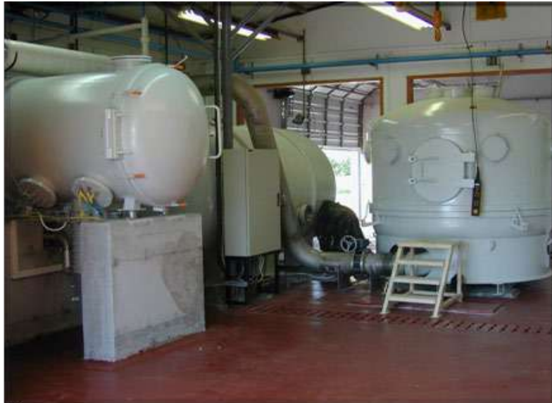
Vacuum chambers for space simulation at Rafael Test Firing Facility
