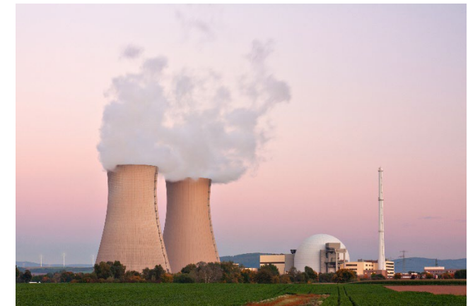
Terrestrial Nuclear Fission Reactor
