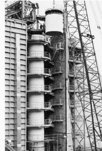
Segment “Stacking” at CSD's ST-9 Static Test Facility
