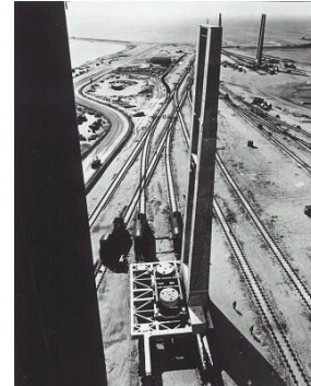
Rail Car for SRM Buildup
