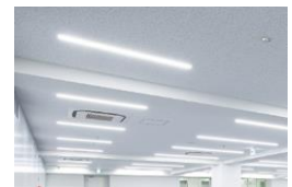
Installation of LED lighting systems
