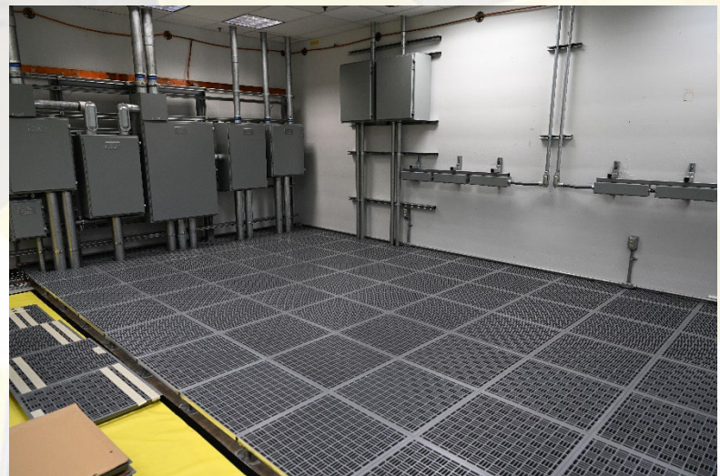
▲ CR1 elevated cable management system.
